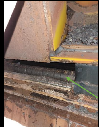
Domite loaf liners during their second 20-week repair cycle
