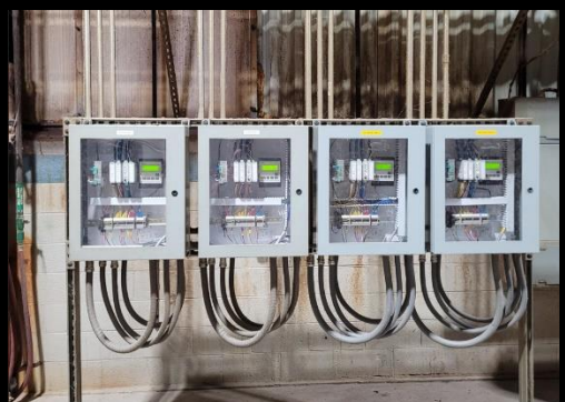
Interface panels into existing BMS
